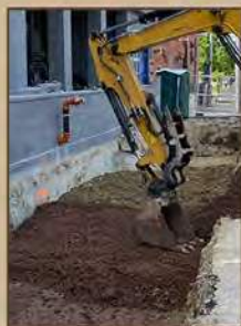
CU-STRUCTURAL SOIL® PORTSMOUTH
