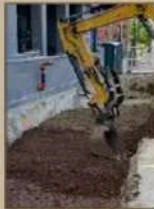
CU-STRUCTURAL SOIL® PORTSMOUTH
