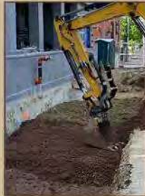
CU-STRUCTURAL SOIL® PORTSMOUTH
