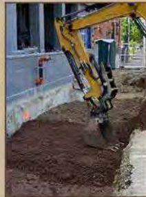
CU-STRUCTURAL SOIL® PORTSMOUTH
